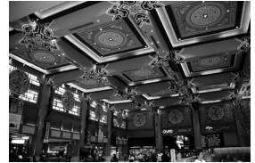
Figure 3 China Court Coffered Ceiling
